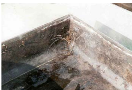
DETAIL OF THE CONTAINERS: THE ROOTS OF THE PLANTS HAVE NOT NOTCHED AND/OR PERFORATED THE NOVAGLASS MEMBRANE
